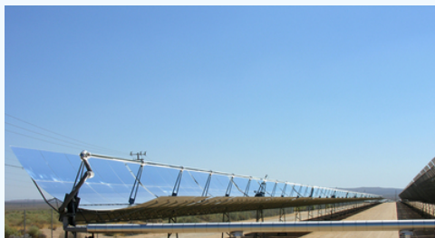
Figure 25.7.5: Parabolic trough collectors are used to generate electricity in southern California. (credit: kjkolb, Wikimedia Commons)
